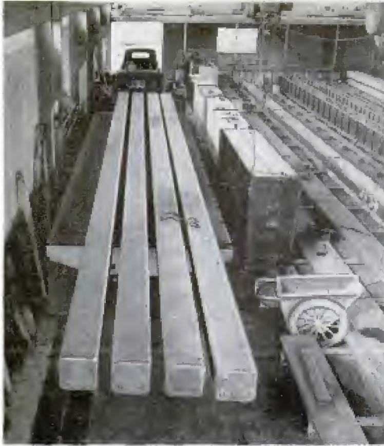
Four 50-foot lengths of piling made of prestressed concrete are shipped by truck, like other materials, to building site
